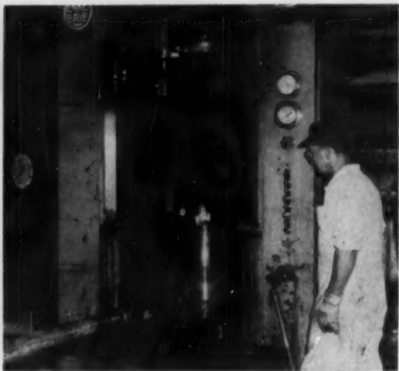
Following rough machining, shells are put in the Surface rotary furnace at rear. Shell noses are brought to 1850° F for nosing (foreground). Mechanical arm picks shells from the nosing press and loads them into cars for the trip to heat treating
